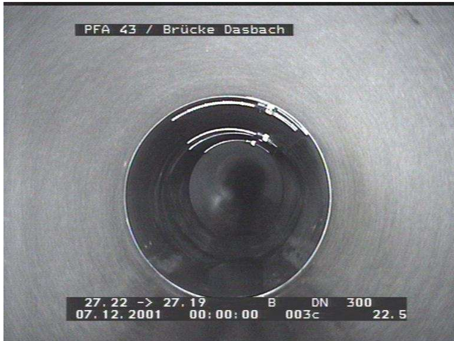
Figure no. 4 – Repaired sewage pipe
